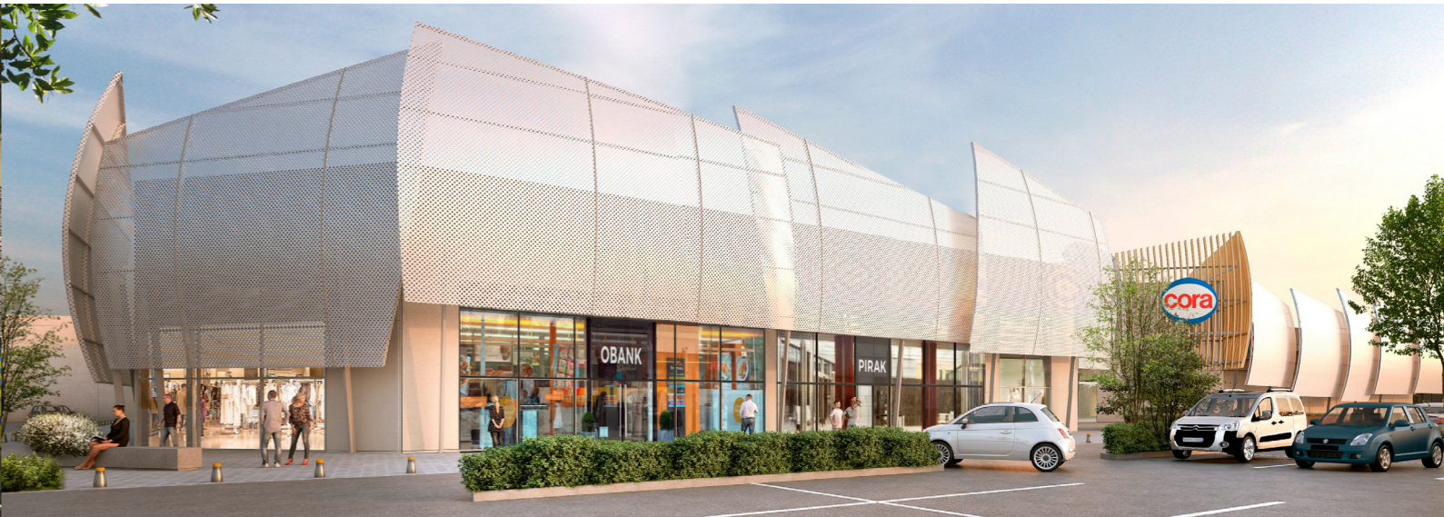
CENTRE COMMERCIAL RENNES-PACÉ (35)
