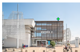
Extension-rénovation Shop'in Pacé (Rennes)
